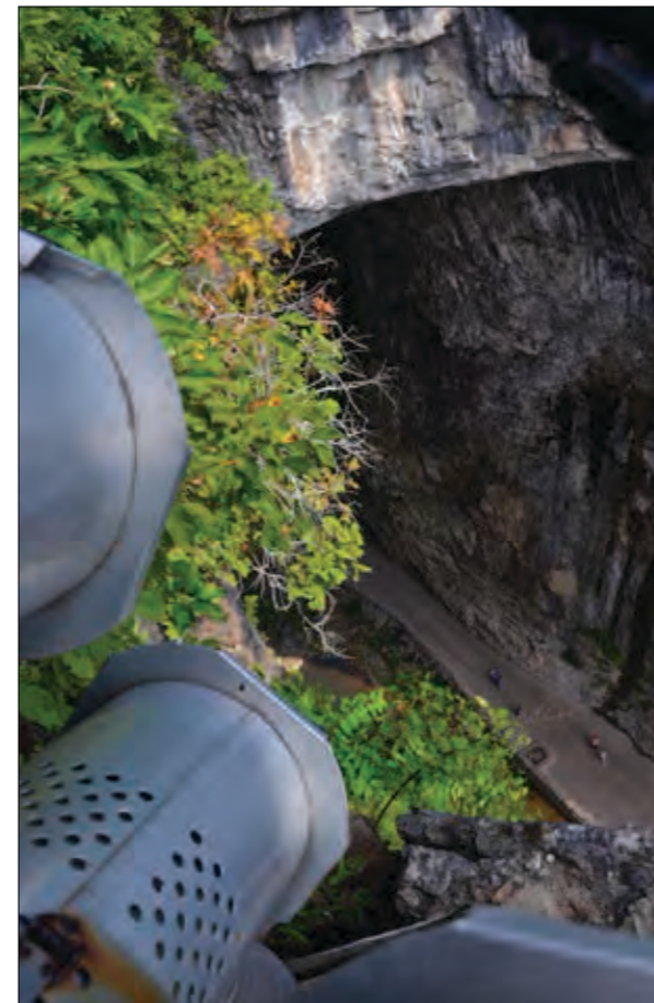
Left: View from the top of the Bridge looking down on Cedar Creek.
