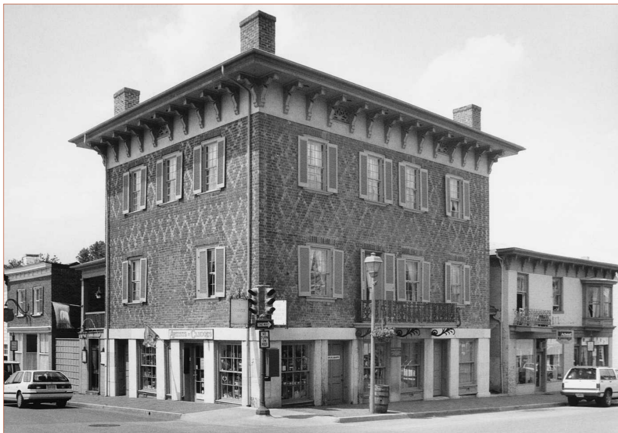
The Alexander-Withrow House at the northwest corner of Washington and Main Streets, after restoration. Note the distinctive diamond-shaped brick pattern. Photo courtesy of the Virginia Department of Historic Resources.
