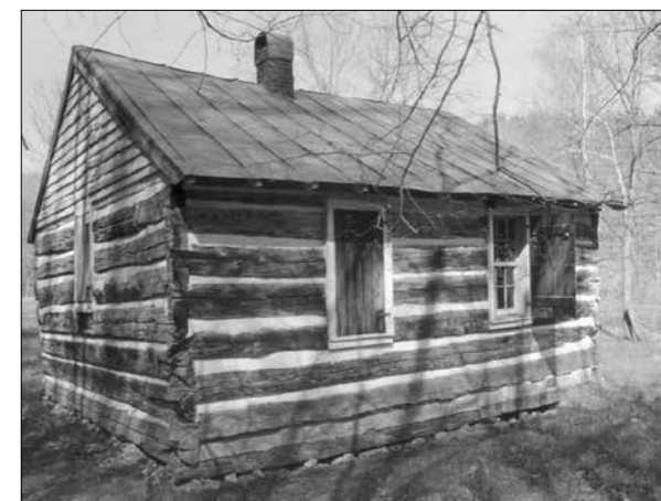
Hamilton School, 1909 (top) and 2002 (DHR photo). Note that in the older photograph, the window has fifteen panes; in the newer photo, twelve.
