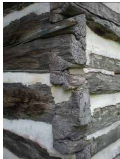
Notched corner logs, Hamilton Schoolhouse.
