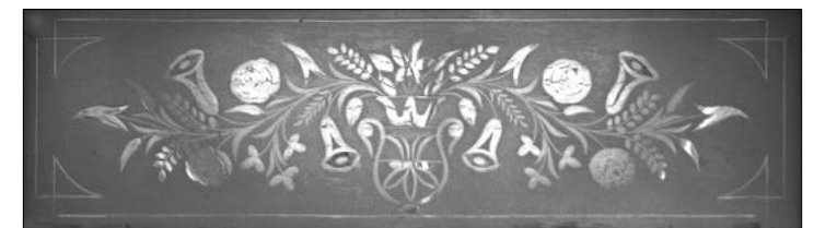
Etched-glass transom window over the front door
