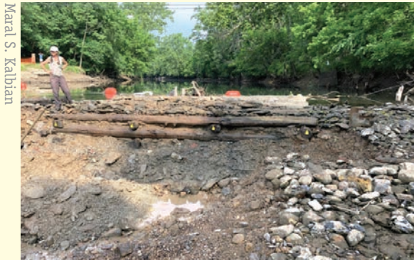
Crib dam uncovered at Jordans Point in 2019
